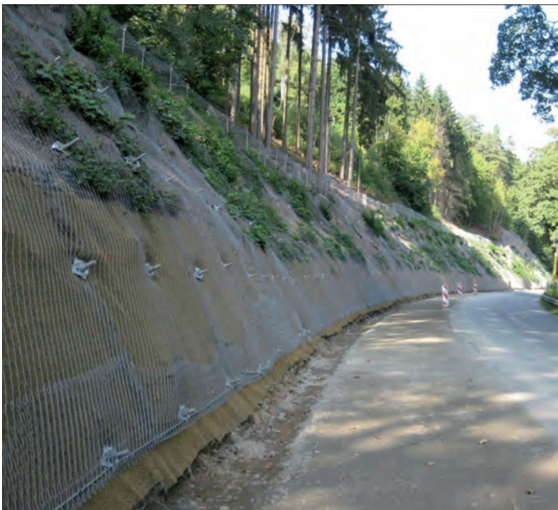
Fig. 4: Exemplary slope stabilisation with high-tensile wire mesh, soil nailing and erosion control mat [5]
