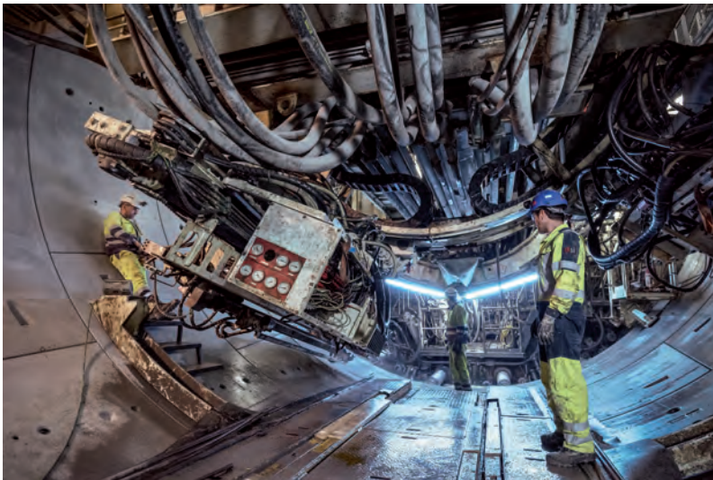
Fig. 9: Regular maintenance and repair of the machines and their components are a prerequisite for consistently high advance rates in the complex Norwegian hard rock.
