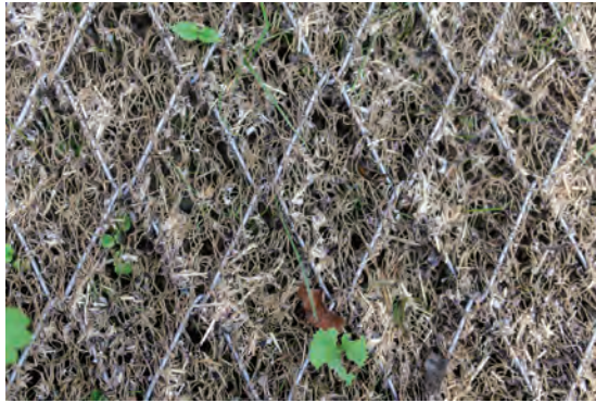
Fig. 14: Erosion and greening mesh made of high-tensile steel wire and mat consisting of three-dimensional polypropylene textile after hydroseeding
