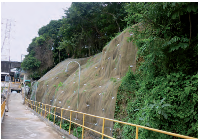
Fig. 11: Rock slope in Miraflores, Panama, secured with mesh and erosion control mat
