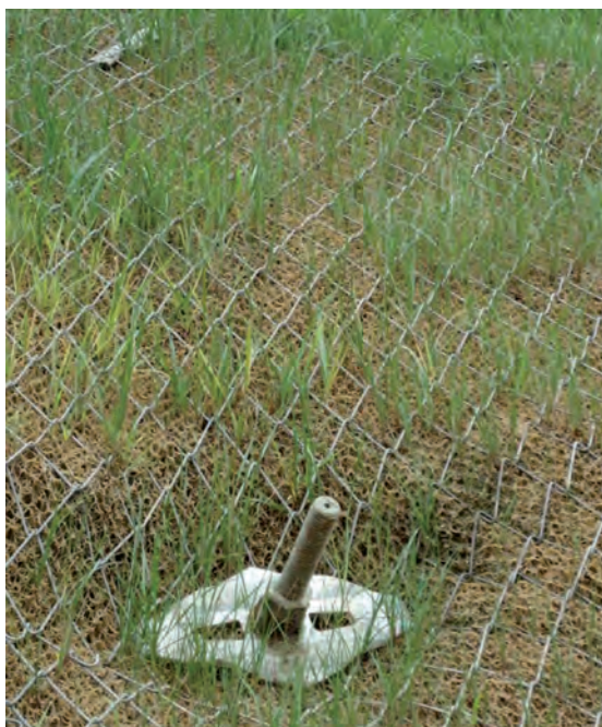
Fig. 10: Erosion control mat Tecmat [8], high-tensile steel wire mesh [6] and soil nailing
