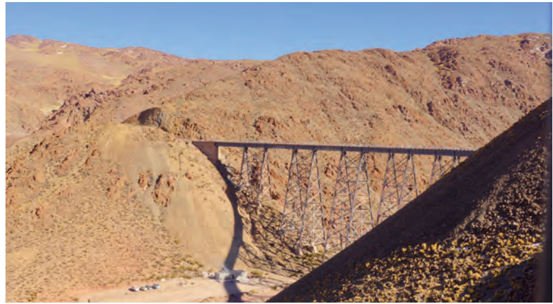
Fig. 4: Viaducto Polvorilla – a 223 m long steel framework construction with 63 m the highest viaduct in South America
