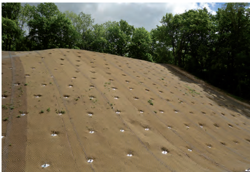
Fig. 13: Uniformly profiled slope in loose rock with close-fitting erosion control mat
