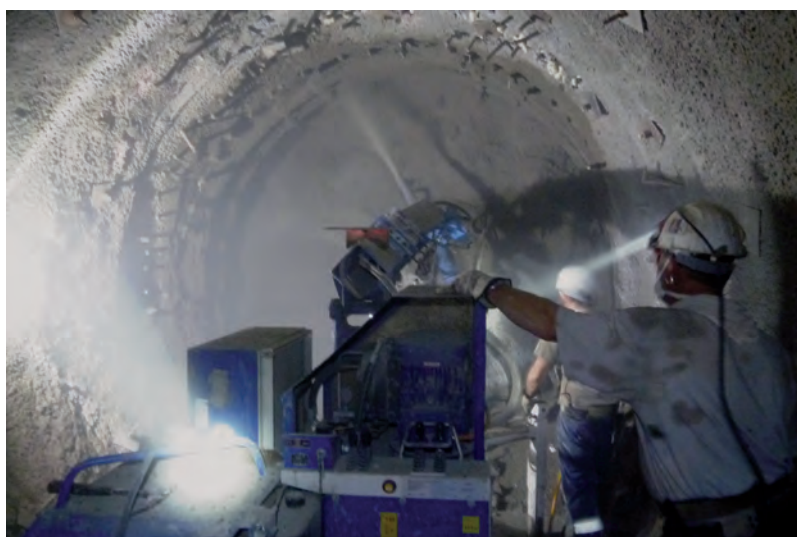
Fig. 8: Shotcrete manipulator Type Meyco Oruga Source: www.epircoc.com
