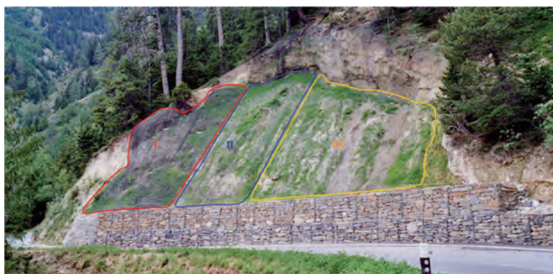
Fig. 7: Test areas in Switzerland for evaluating different erosion control mats on a steep slope
