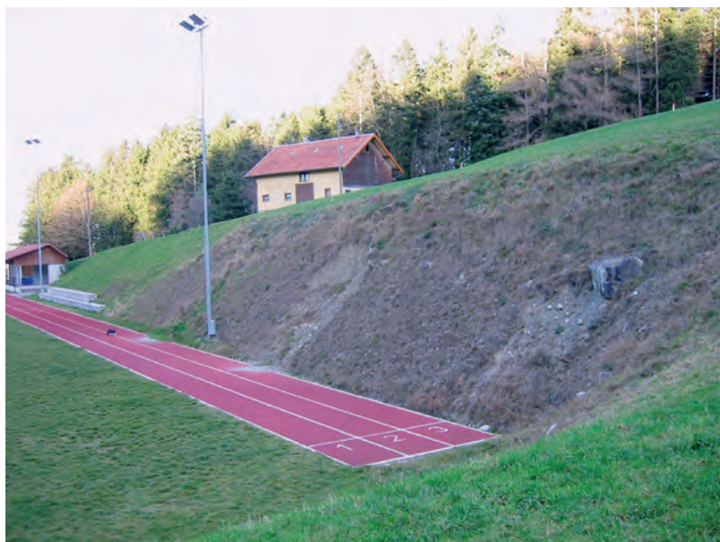
Fig. 1: Ad hoc slumping on a slope in the grounds of a sports facility Source of images: Geobrugg AG
